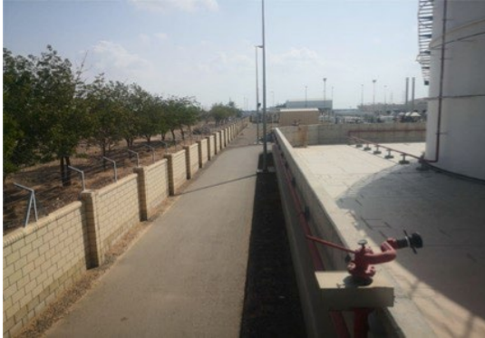
Figure 4: Wall Surrounding the Site
